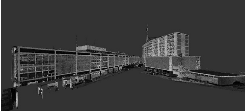
Perth Police Station, Australia
